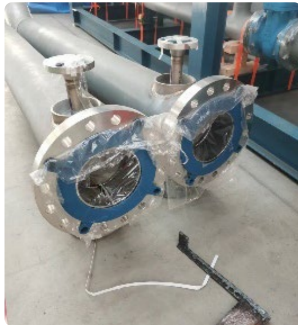
Sealing Material Replacement
